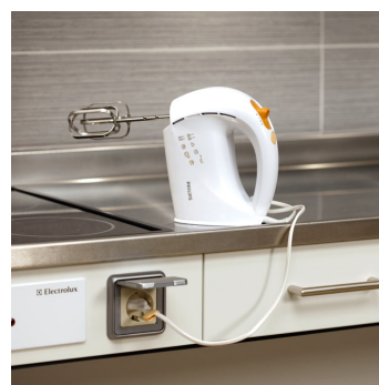
Power sockets can be integrated in the front so that they are easily accessible from a sitting position.
