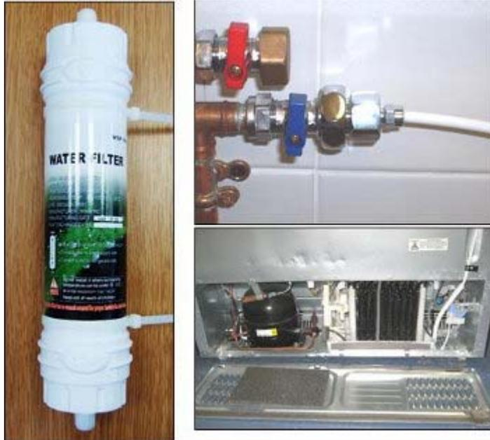
The pipe from the filter is on the right-hand side and is connected to the valve as shown. The other pipe on the left is the water supply from the valve up to the ice maker and this should not be disturbed. The grey hose is the water supply that leads to the chilled water tank inside the bottom of the fridge compartment. This should also be left alone.
